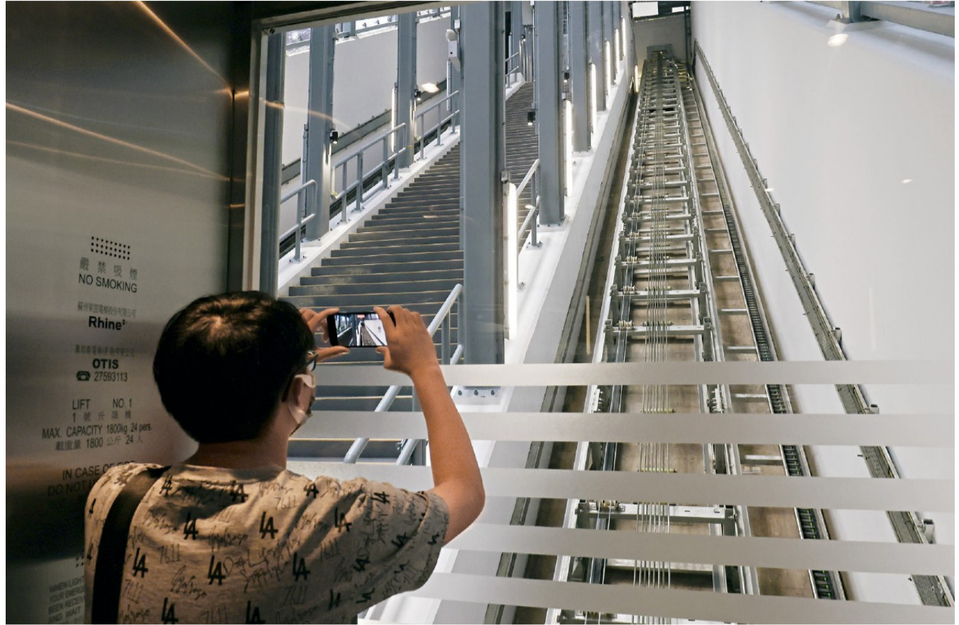
A passenger takes a photo while riding the first lift built on the hill at Kwai Chung Estate yesterday, its first day of public operation. The system consists of two coaches that can hold up to 24 people
